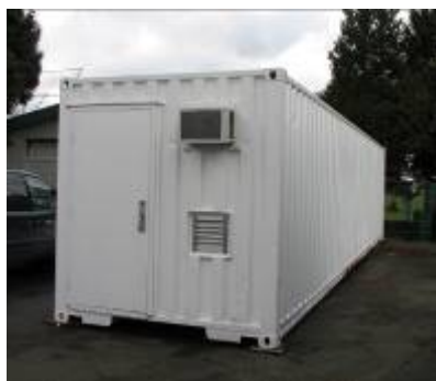
Fig. 1. Insect rearing facility modified from a 40 ft marine transport container.
